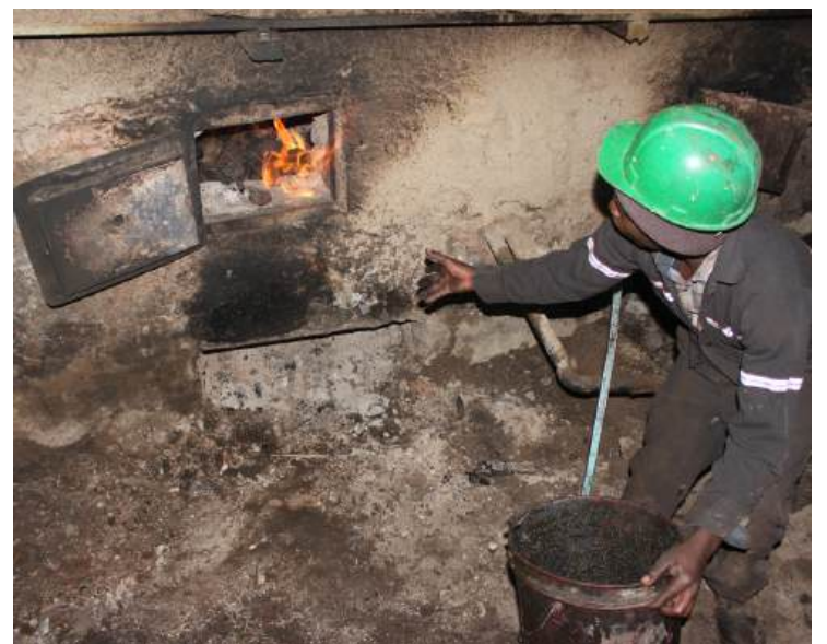
A worker feeds briquette into a furnace /KNA
