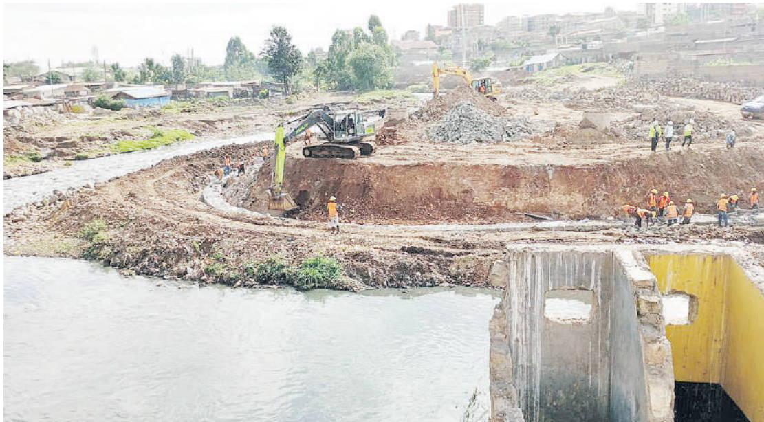
Ongoing works at Lucky Summer /HANDOUT
