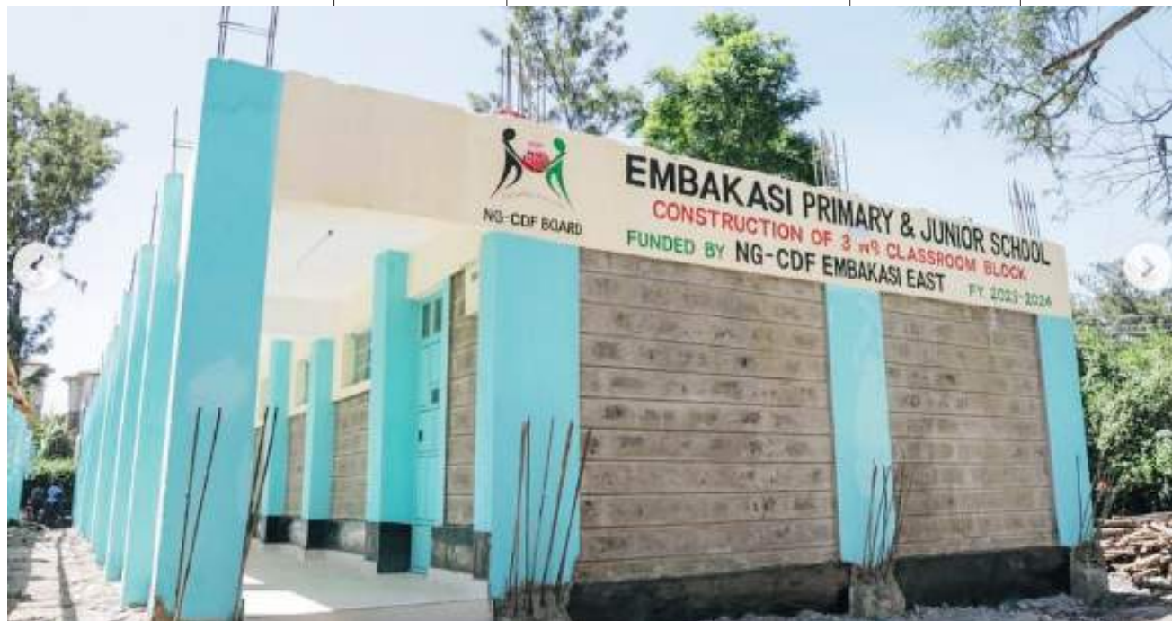
Classrooms under construction at Embakasi Primary and Junior School /HANDOUT
