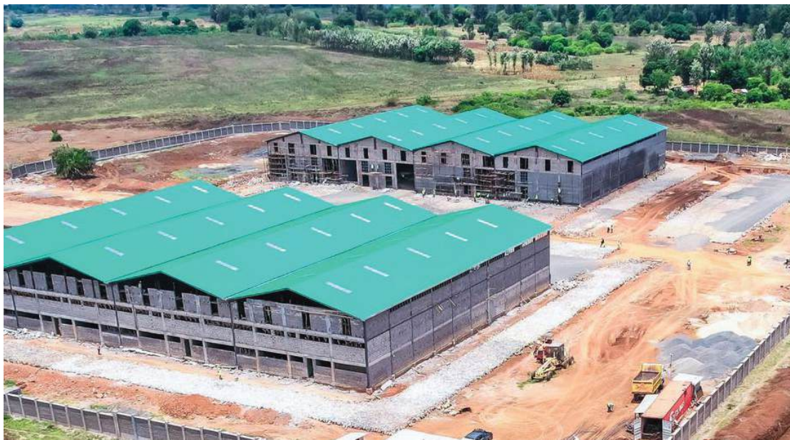
Sagana Industrial Park in Kirinyaga county/FILE
