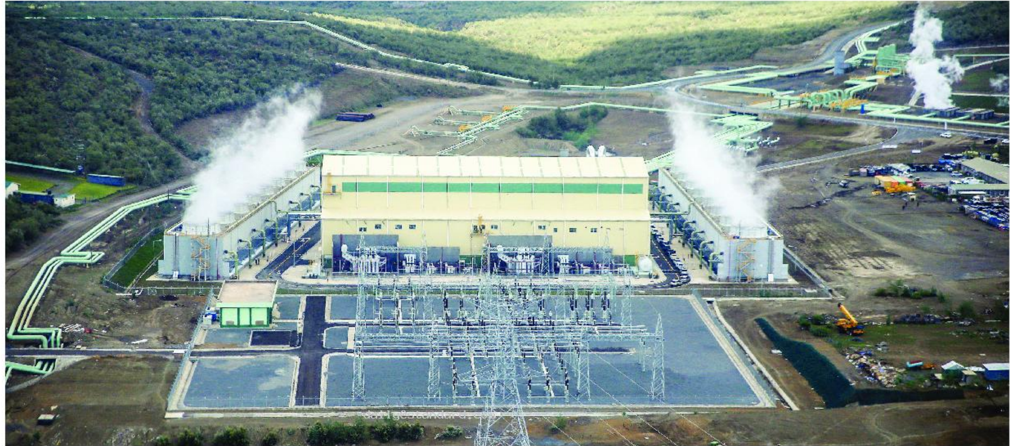
Aerial view of the 140 megawatt Olkaria IV Geothermal Power Plant in Naivasha sub-county. [File, Standard]
