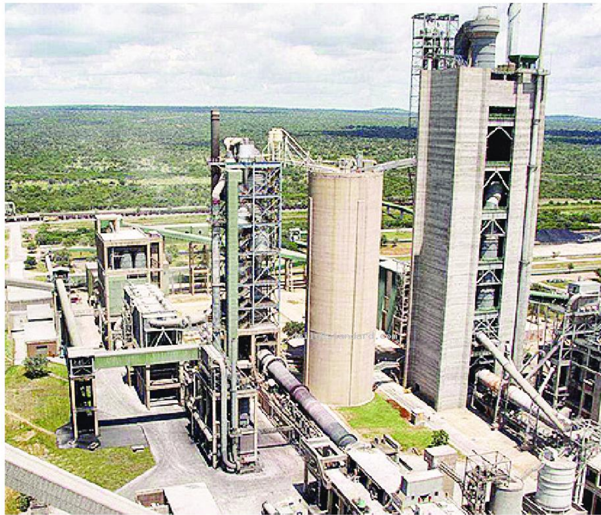
The East Africa Portland Cement factory. [File, Standard]
