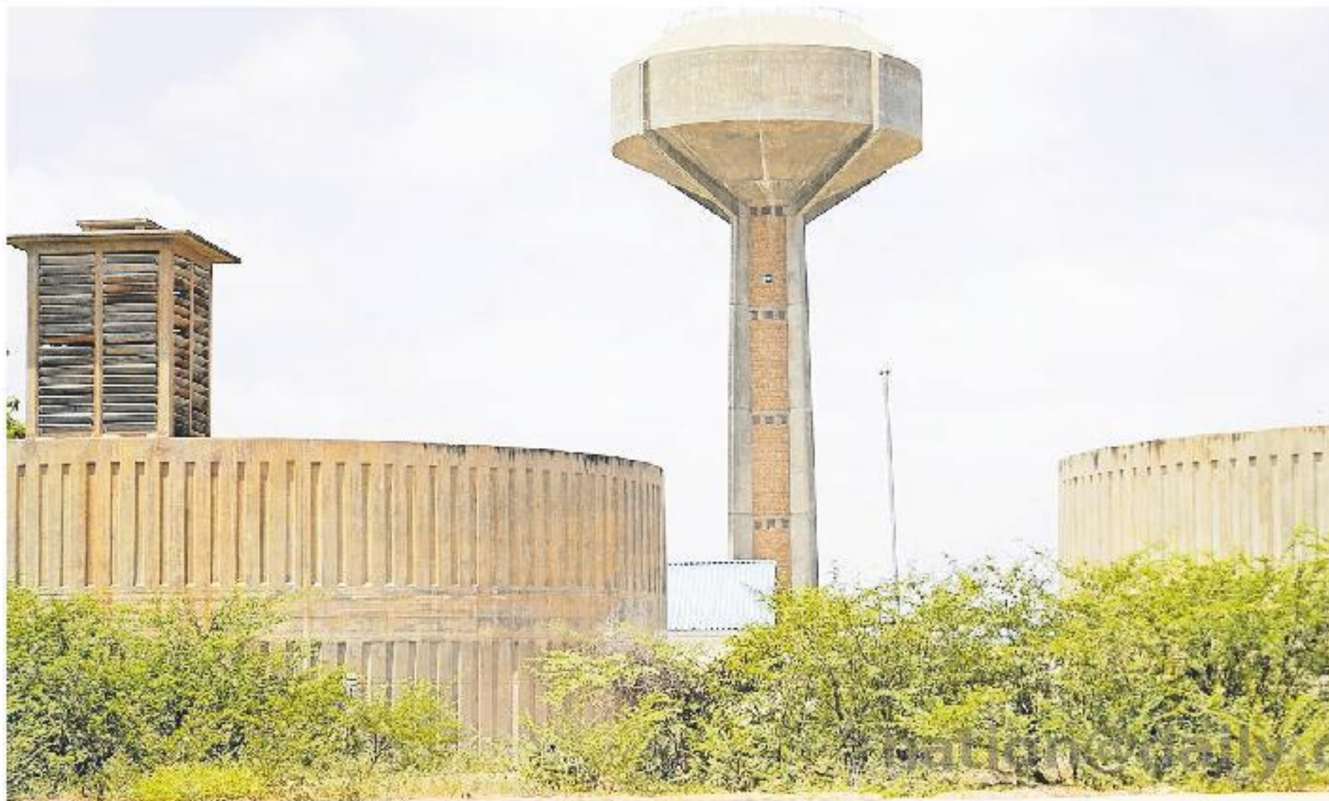
The multimillion-shilling water supply tower in Bura, Tana River County. STEPHEN ODUOR | NATION
