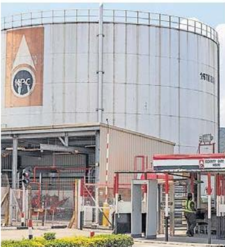
The Kenya Pipeline Company depot in Nakuru on November 22, 2024. BONIFACE MWANGI | NATION
