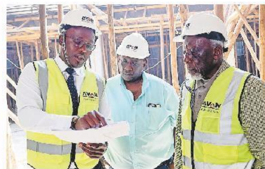
From L-R: Chief Executive Officer Felix Kimanthi, Investment Committee Chairperson Patrick Wamae and Chairman Olympia Capital Holdings PLC, Dr Chris Obura, inspect the Avon Arcade project, a commercial development under the group's real estate arm. The project, which is located along Enterprise Road in Nairobi, will cater to small-scale traders.
