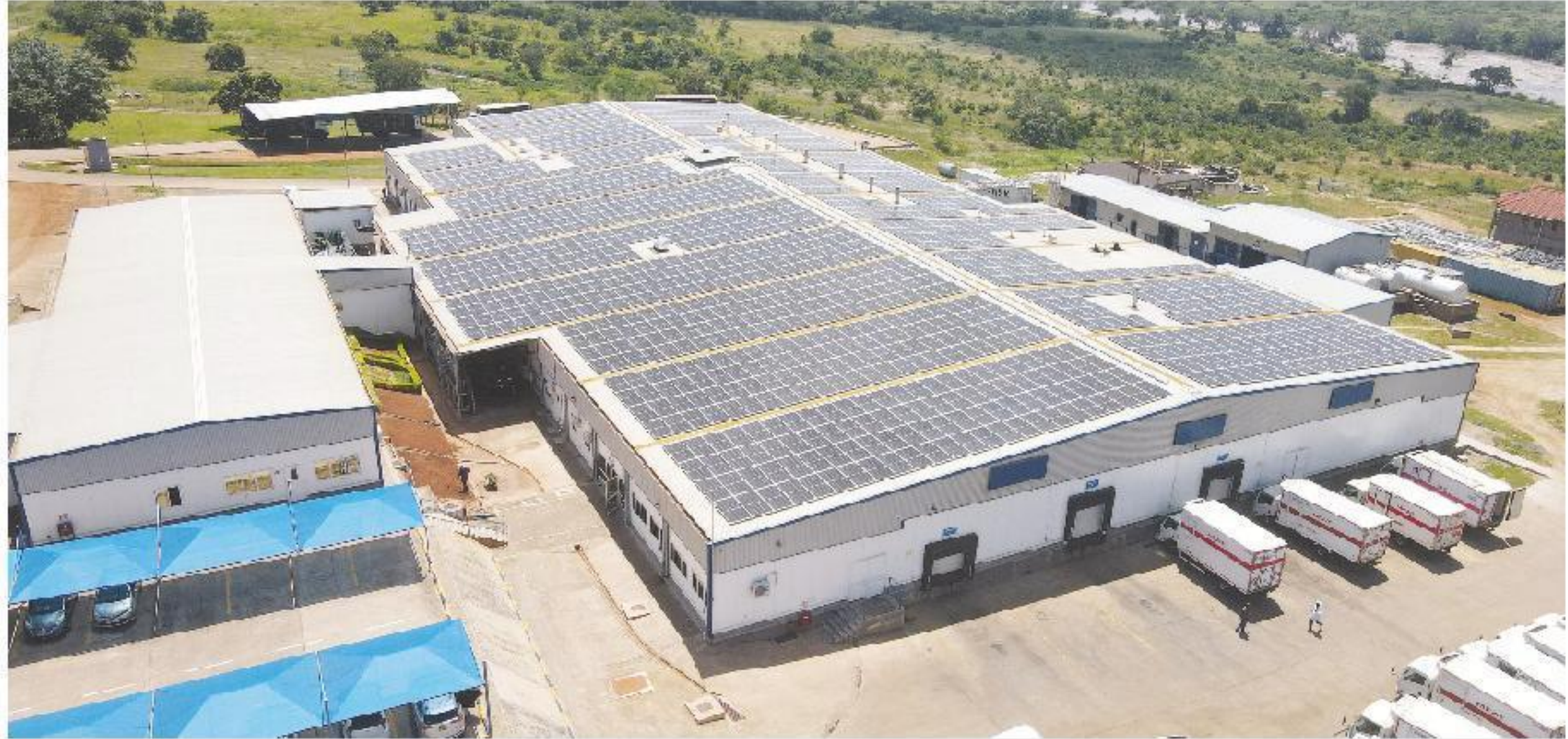
Solar panels at the Kenchic processing plant.
