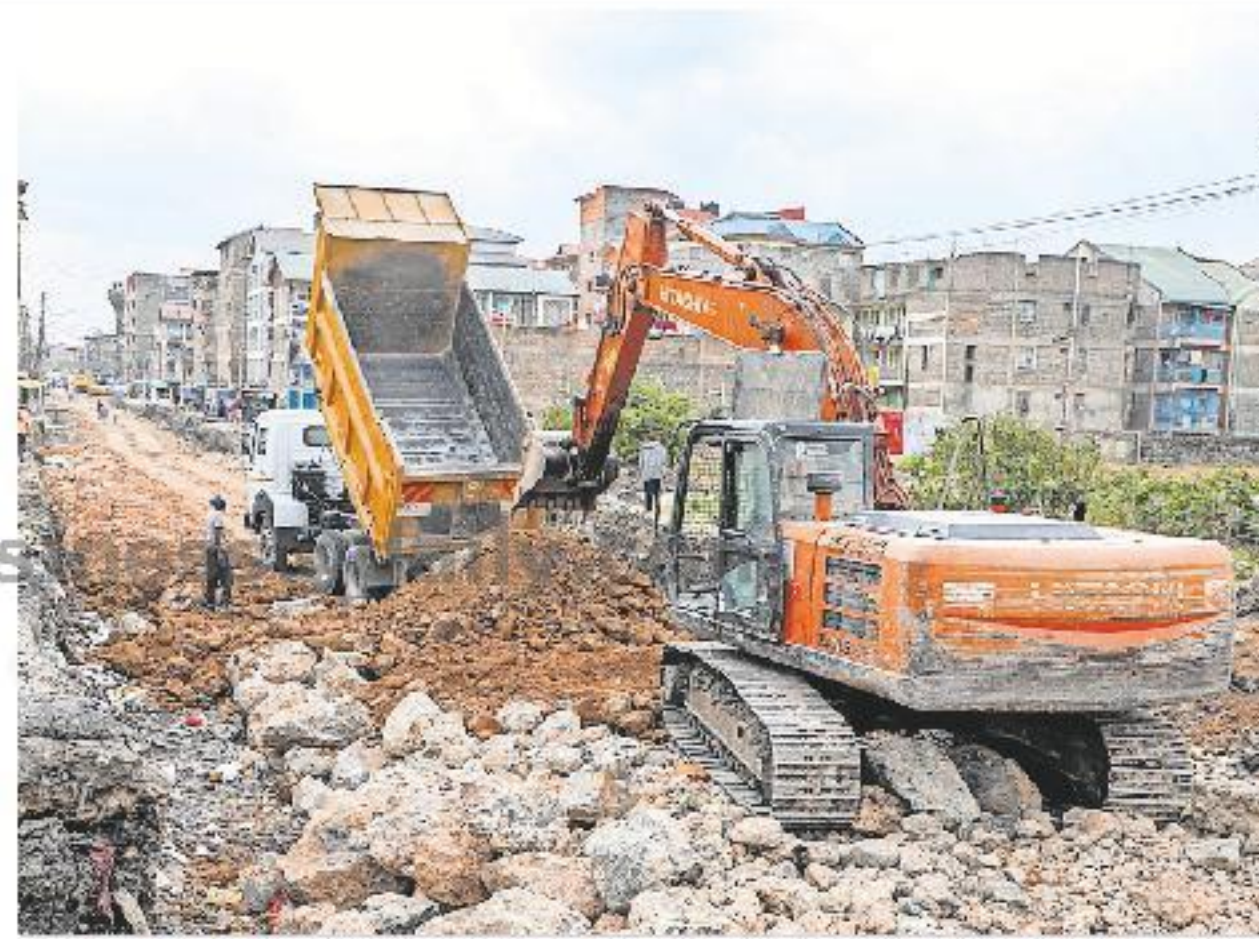
Rehabilitation works on a road in Nairobi's Embakasi West. DENNIS ONSONGO
