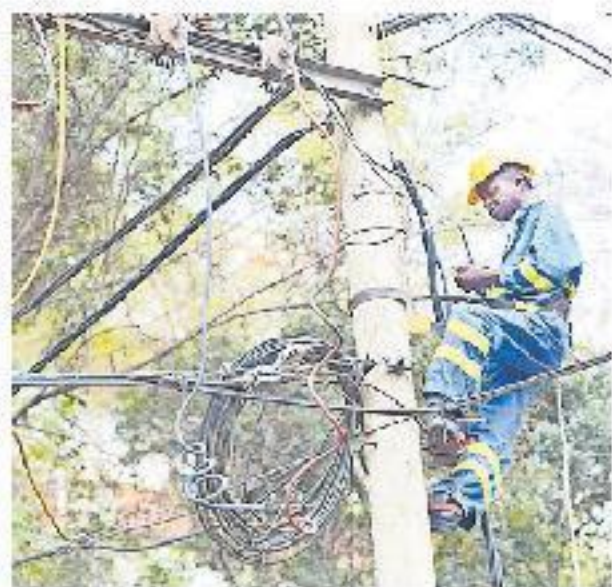
A Kenya Power employee conducts repair and maintenance works.
