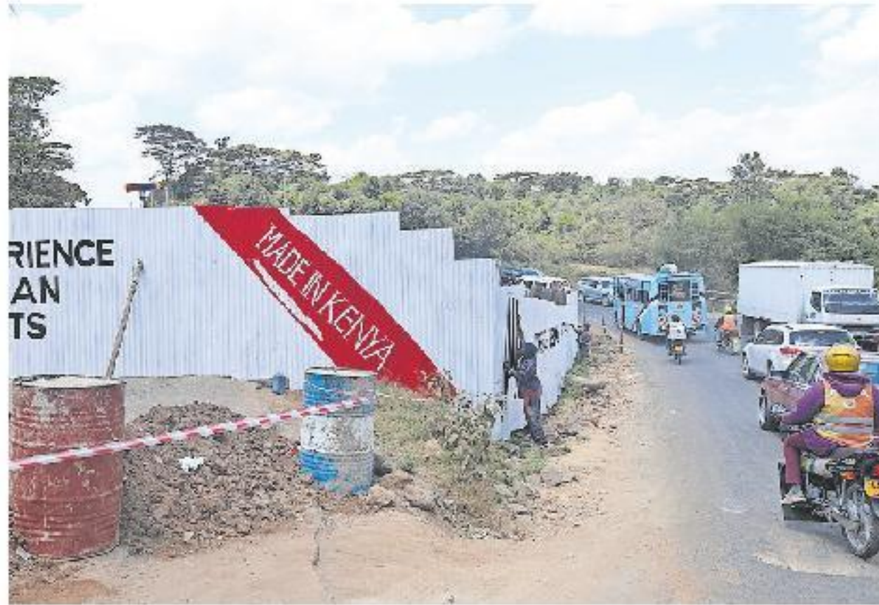
Construction works along Magadi Road in Nairobi on September 10. EVANS HABIL
