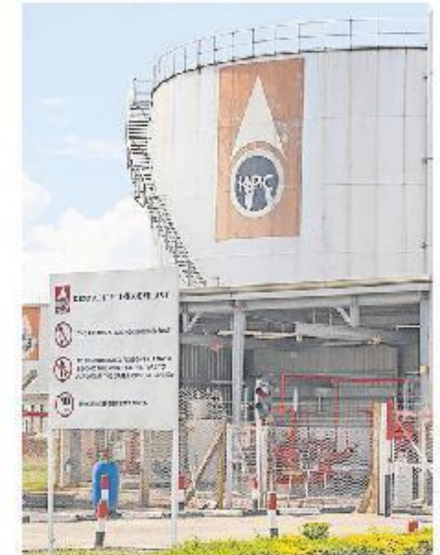
The Kenya Pipeline Company depot in Nakuru.
