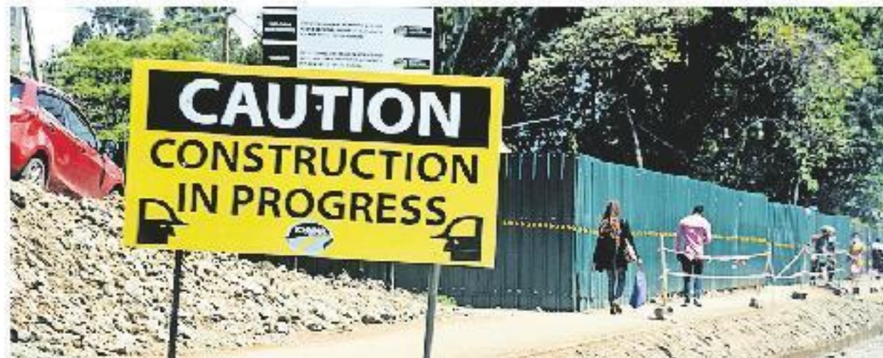
Construction work at T-Mall junction on Lang'ata Road, Nairobi in 2020.
