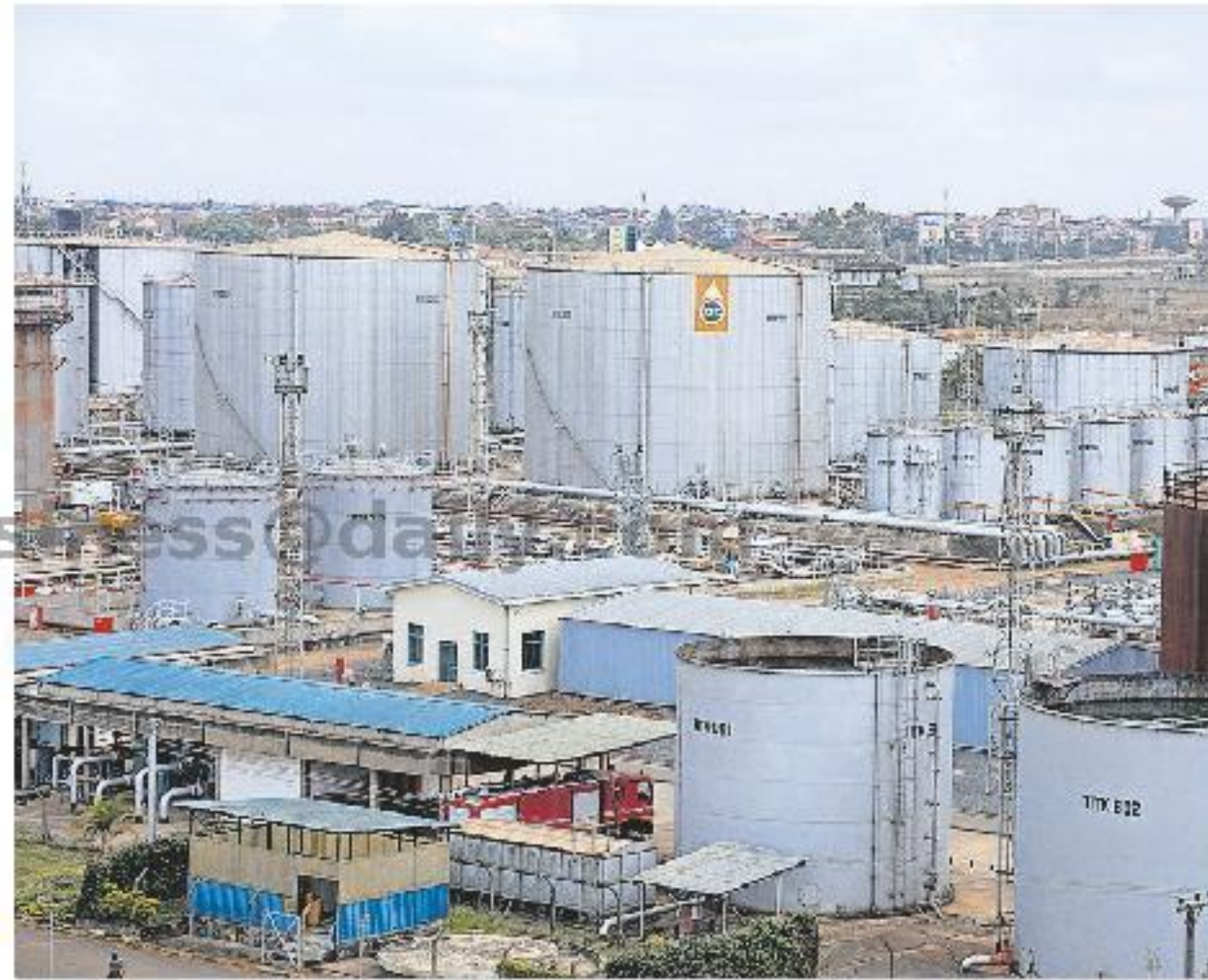
Kenya Pipeline Company petroleum storage facility in Industrial Area, Nairobi. FILE
